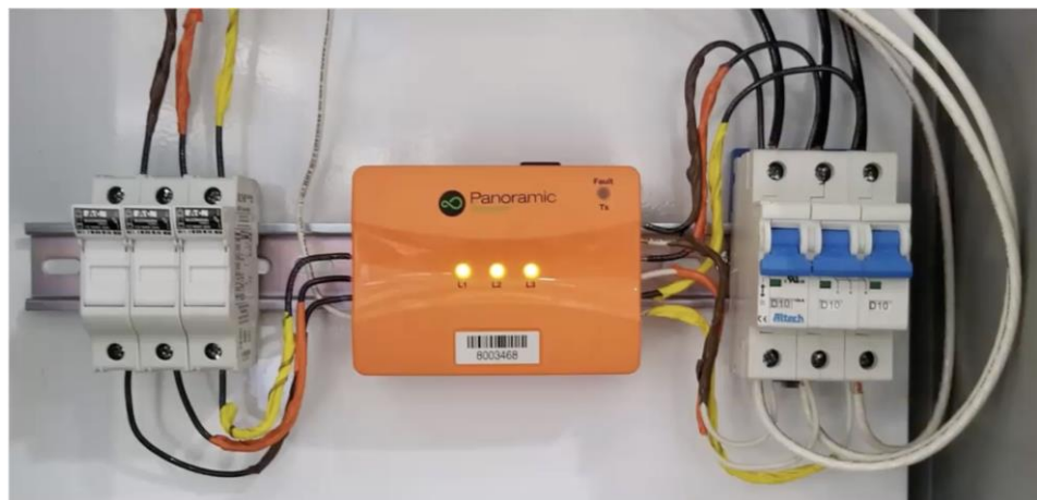
PAN-42 installed on a DIN rail
